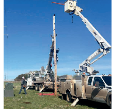
An Oahe Electric crew converts overhead lines to underground for enhanced reliability.
