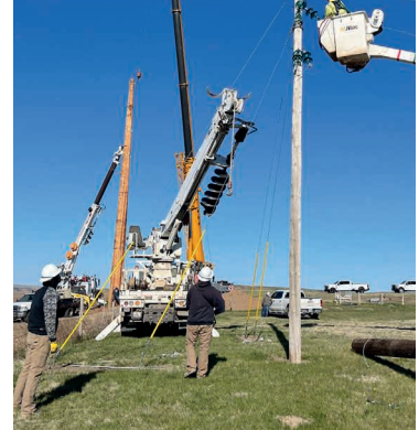
An Oahe Electric crew converts overhead lines to underground for enhanced reliability.
