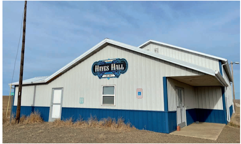
For a few nights every year, Hayes Hall gets packed to standing-room only. West Central Electric Cooperative provides the hall's electrical power and is an annual sponsor of the Hayes play.
