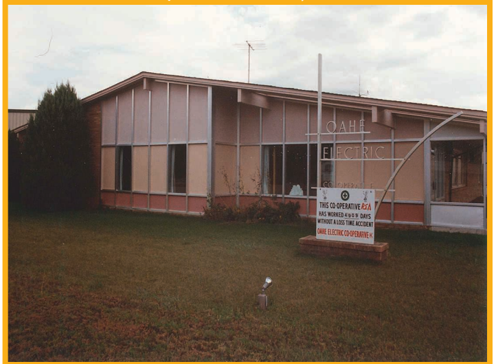
The old Oahe Electric headquarters back in the day.
