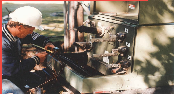
Rodney at work as a young lineman in the field.
